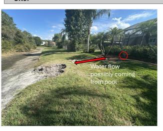
Pipe found on outside of screen where I assume they are emptying their pool from. You can see bare spots in the yard and some minor washouts occurring near the landscaping bed that lead me to believe there is excessive water flow coming through this area, leading straight to the eroded area.
