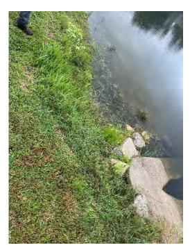
Location 31: Clear overgrown vegitation from around mitered end section to ensure proper flow.
