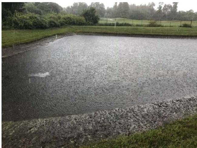
C03 - Excellent condition. The bank is free of any and all nuisance grasses, while the water is clear of algae. Rain fell here during the inspection, but this did not impact the quality of the evaluation.
