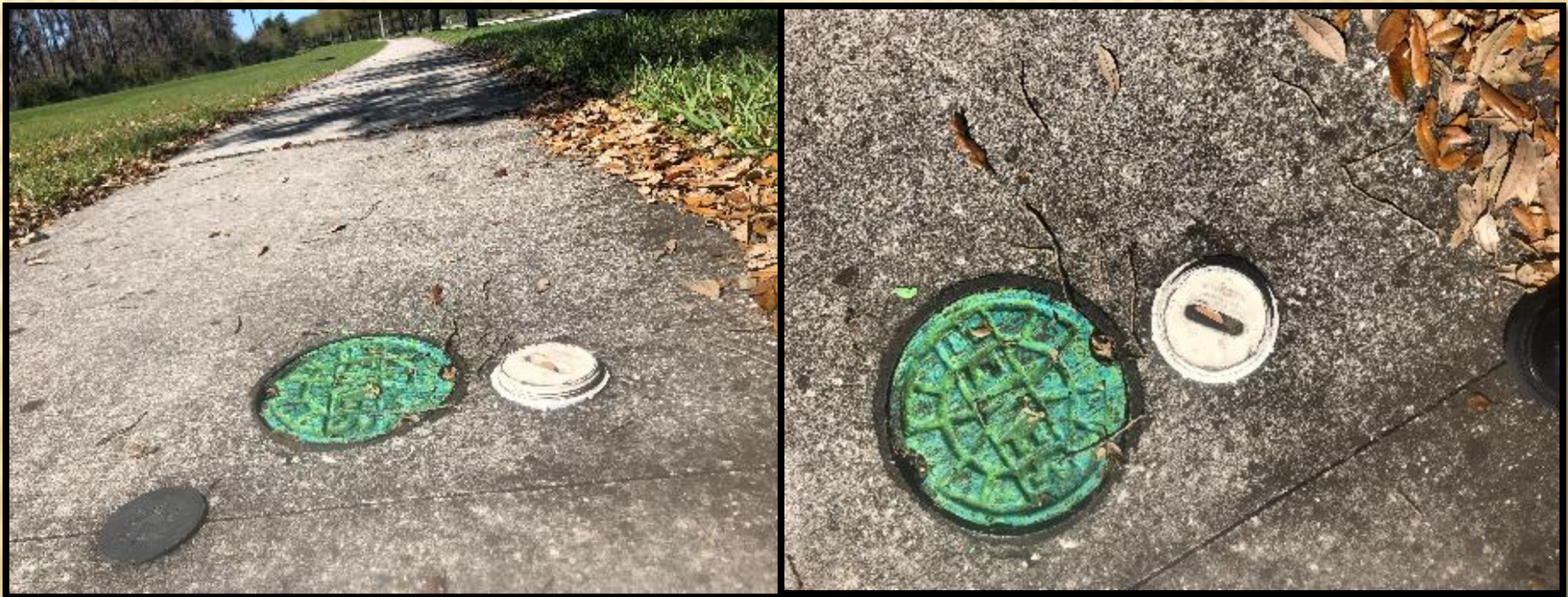
Raised Cap Tripping Hazard North Side of W. County Line Road
