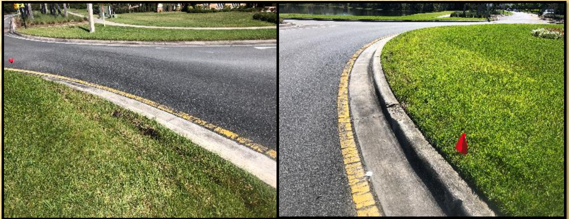
Curb at Rotary Damaged
